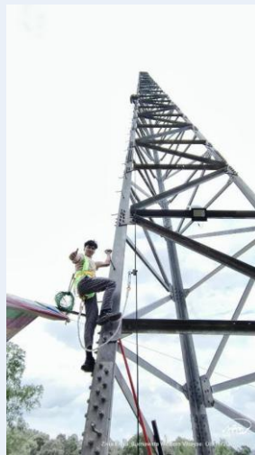
Work on the radio tower
