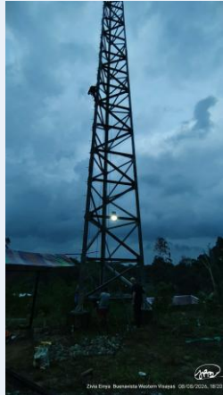
Working on the tower in the cooler evening hours
